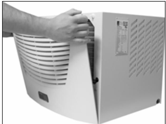
Fig. 22: Release the louvered grille
