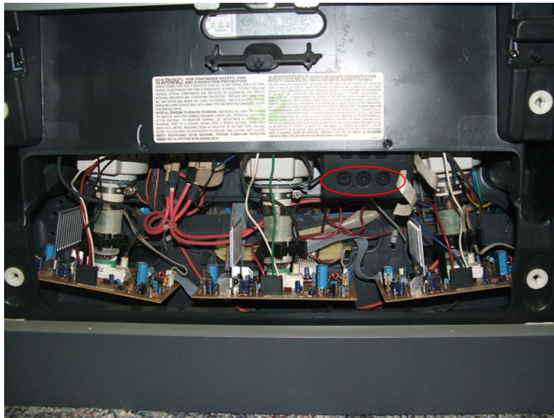
Figure 3: Recess exposed when the lower center panel is removed. Allows access to the CRT Kine socket boards and to the electronic SCREEN and FOCUS controls. Focus controls are circled. They are labeled by color. The SCREEN control is used to set CRT “cutoff” (adjust color temperature). Do not adjust it. Do not touch the tube stems or circuit boards (high voltage electric shock danger)!
