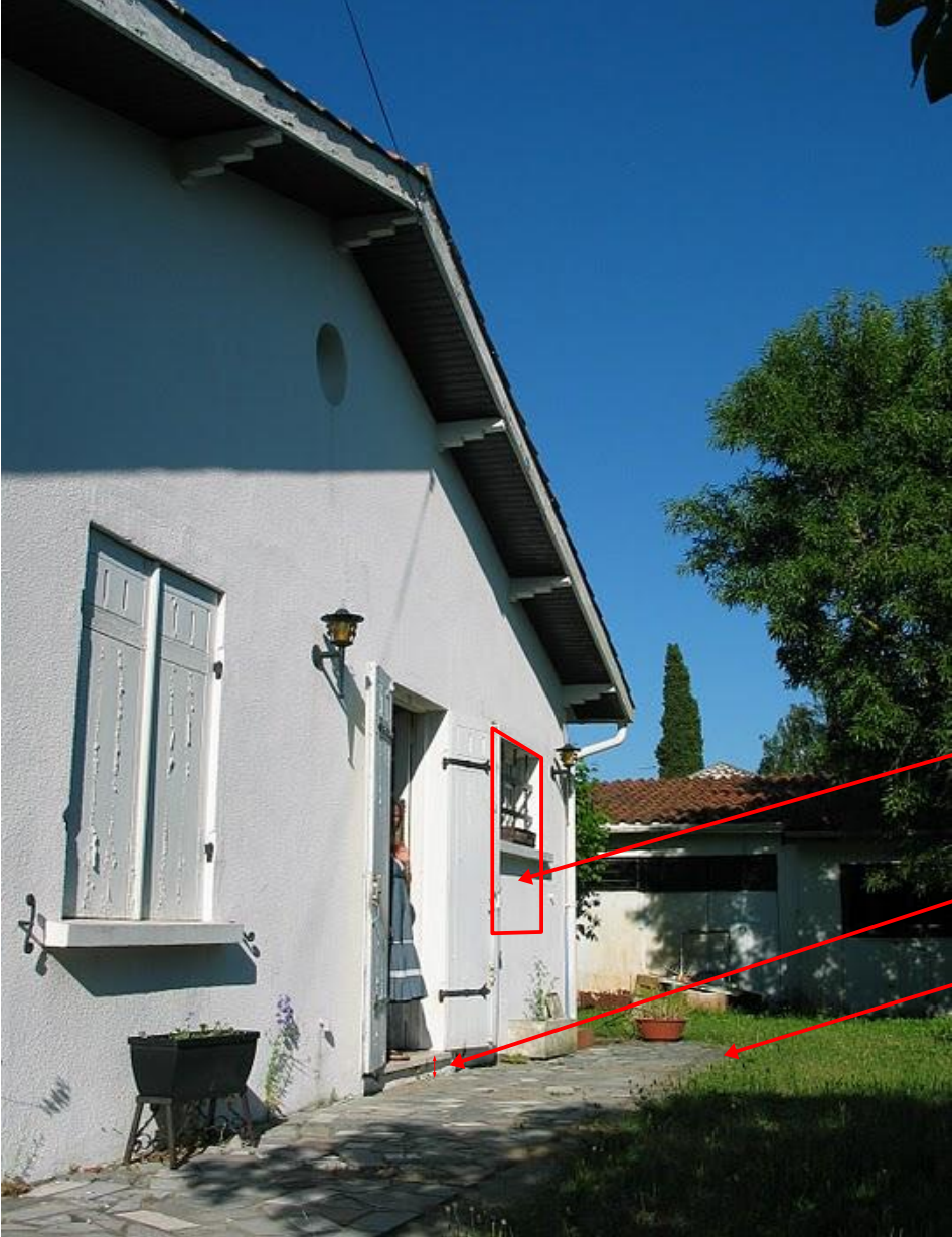
Façade "sud" (SSE)
