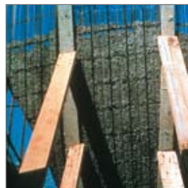
Coffrage double Double formwork
