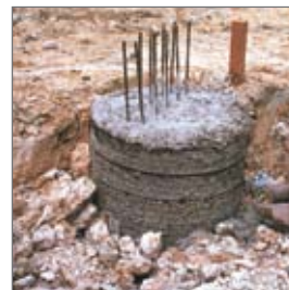
Coffrage cylindrique Cylindrical formwork
