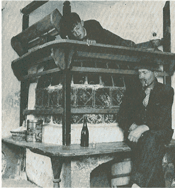
Figure 143 Tile stove with bench and sleeping platform. The stove was photographed in 1942 in the Slovenian region of Yugoslavia, formerly a part of Austria. Photo by Erika Groth-Schmachtenberger.
