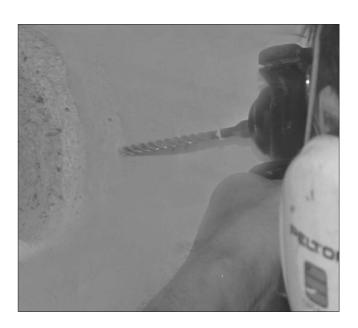
Drill 3x fixing holes and fit 3x wall plugs.
