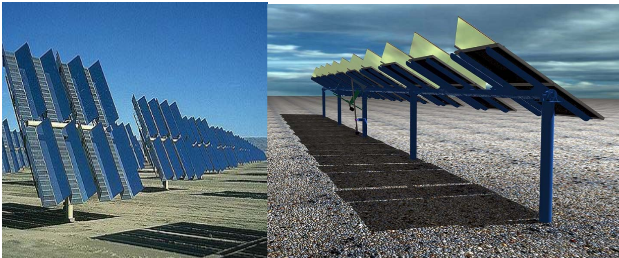
Fig. 1. Left: ARCO photovoltaic plant, Carrisa Plains, near California Valley, CA (1984) 2X side reflectors resulted in severe browning of the ARCO design. Right: artist rendering of proposed geometry. The new 1.5X design (right) allows better convection and radiation cooling. Moving boost mirrors can alter its concentration ratio on hot days. Tracking motors and controls for new design is simpler. The new geometry will be focus of future paper.
